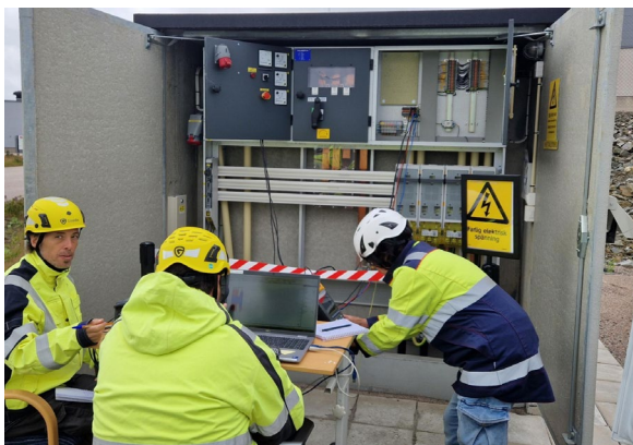
RISE institute & UPV/EHU university's grid impedance and EVCS disturbance measurement team at an EV charging station in Sweden.
